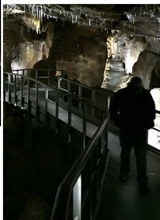
The FRP walkways show very little wear following 10 years of use. Track lights are well concealed within the handrails.
