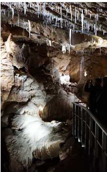
The FRP walkways show very little wear following 10 years of use. Track lights are well concealed within the handrails.
